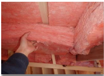
断熱材 (天井) HGW105×3
