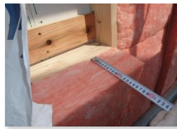
断熱材 (付加断熱) HGW105
